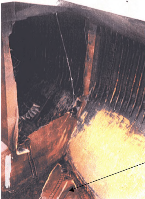
Photograph 1 Collapsed and detached transverse bulkhead
