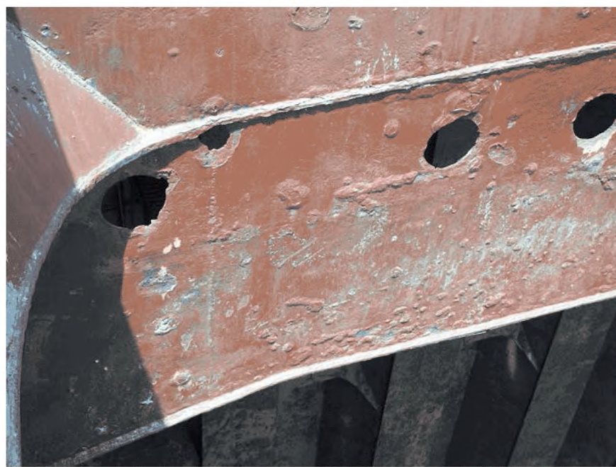
Photograph 2 Heavy corrosion of hatch coaming
